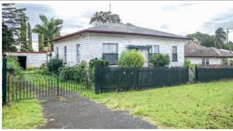
5 Hampshire Street, NORTH TOOWOOMBA
