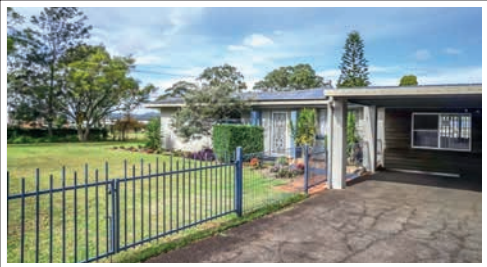
330 North Street, WILSONTON
